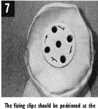
edge of the ceiling aperature and once pinned in place the firehood maybe opened out
