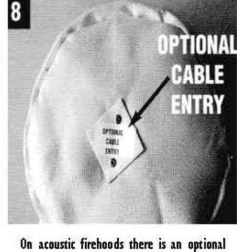
cable entry on the top, normal cable entry is from the bottom of the firehood
