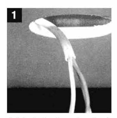
Lead the cable from the transformer through the hole cut for the downlighter fitting
