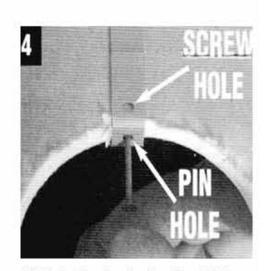
Whilst holding the clip align the pin hole to the ceiling and pin the two together using a supplied fixing pin
