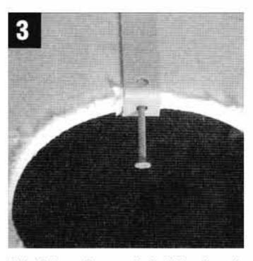
This clip is used to attach the firehood to the ceiling
