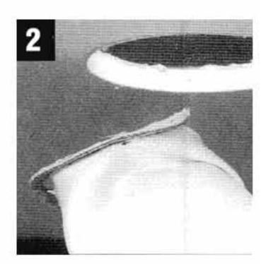
Squeeze the cover to reduce its size and slot it through the hole (retaining a grip on the clips throughout the process)
